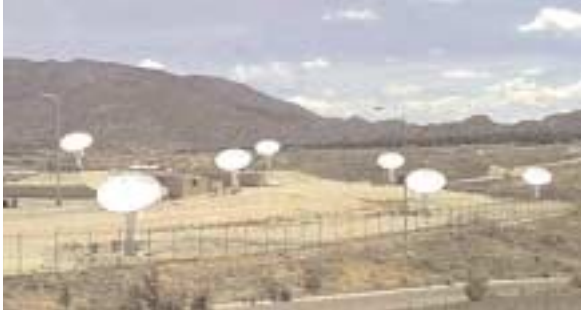
ANTENNA FARM, part of new space-to-ground communication path for NUDET detection system.
