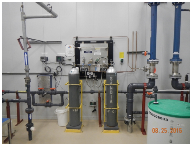
Figure 3-8. SNL/TTR water treatment facility carbon dioxide pH adjustment system
