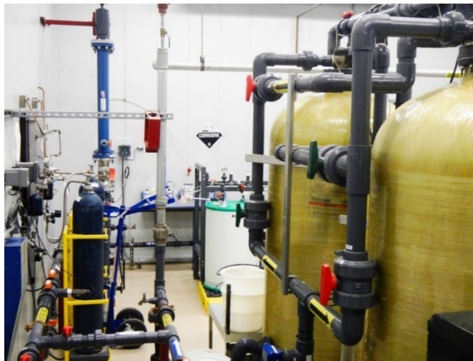
Figure 3-7. SNL/TTR water treatment facility arsenic removal system
