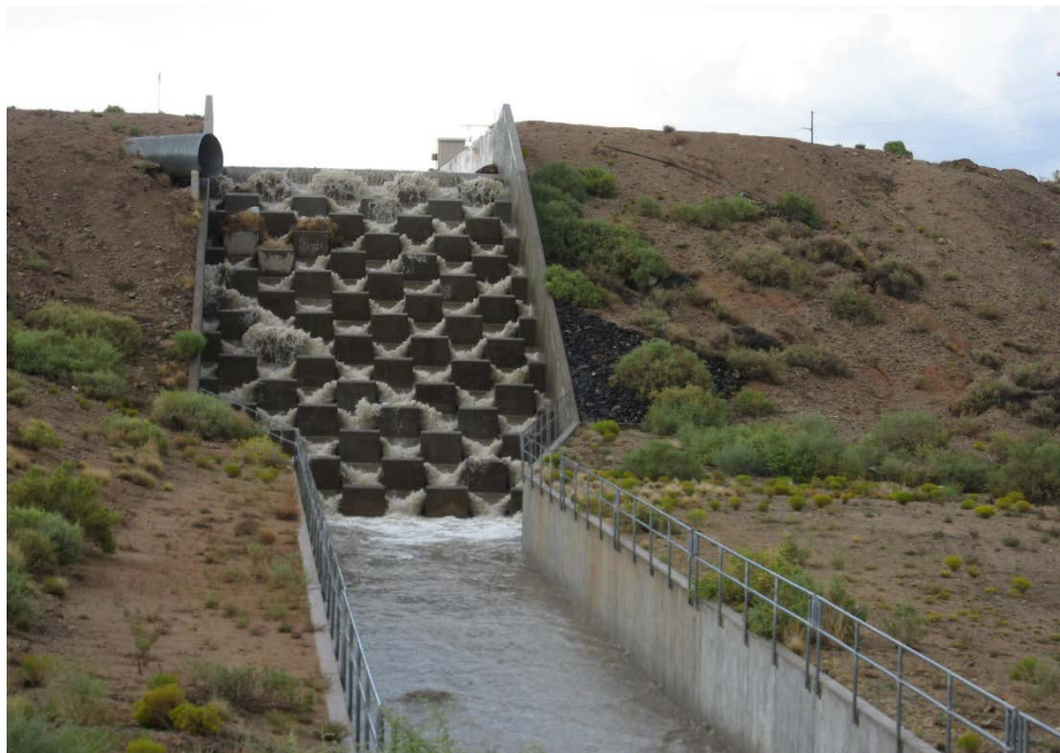
“Dragon’s teeth,” stormwater energy dissipator
