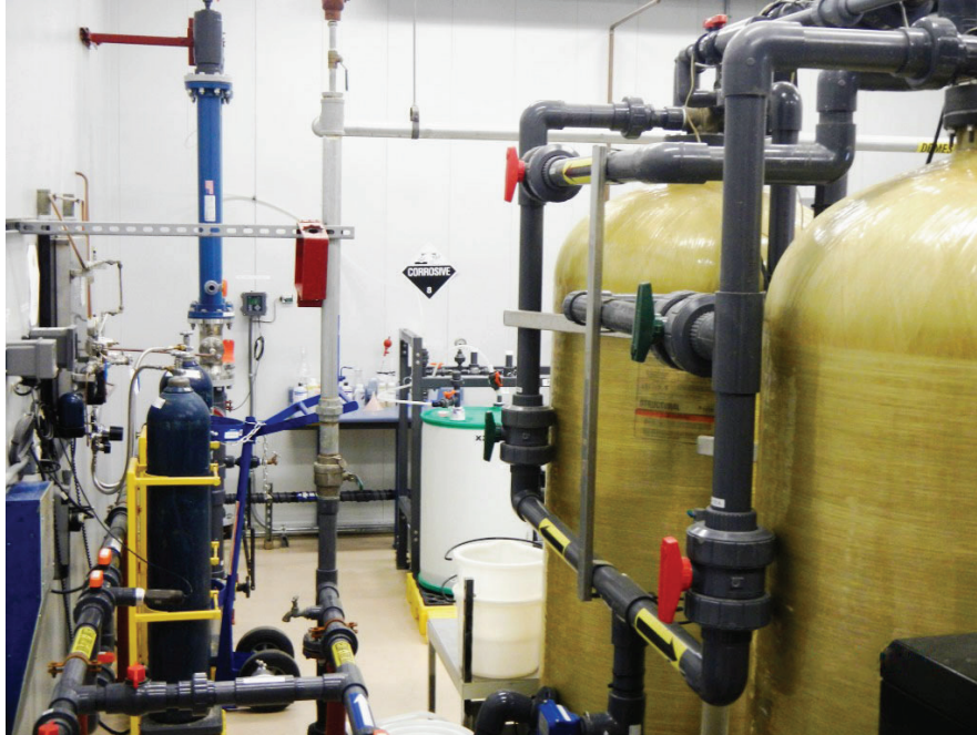
Figure 3-8. SNL/TTR water treatment facility arsenic removal system
