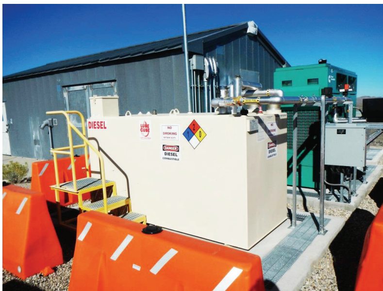
Figure 3-1. SNL/TTR diesel fuel tank (1,000 gal) at Building 24-51
