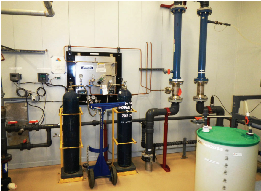
Figure 3-9. SNL/TTR water treatment facility CO 2 pH adjustment system
