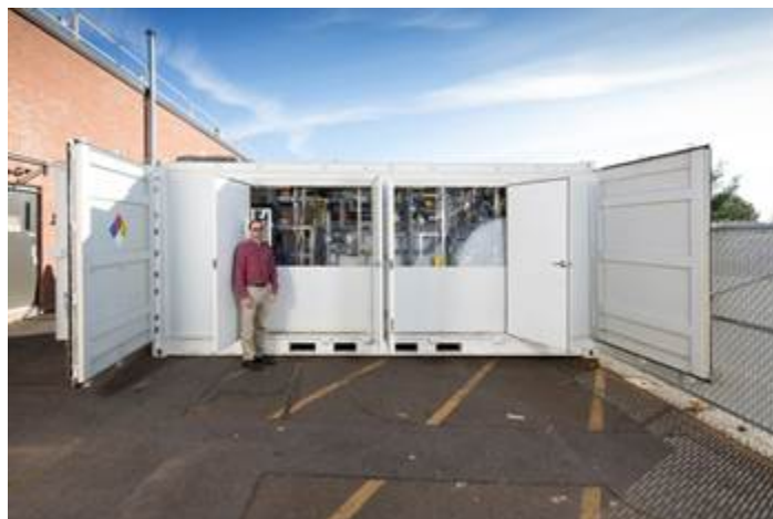
Figure 17: Vanadium redox flow battery [13].
