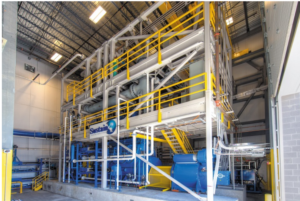
Figure 12: SustainX 1.65 MW isothermal CAES.
