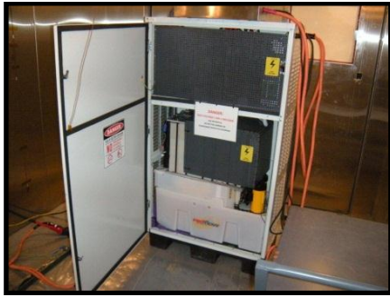
Figure 3: Redflow Zinc-Bromide Battery Module (ZBM) within a System Development Kit (left) and within a demonstration residential unit R510US (right)
