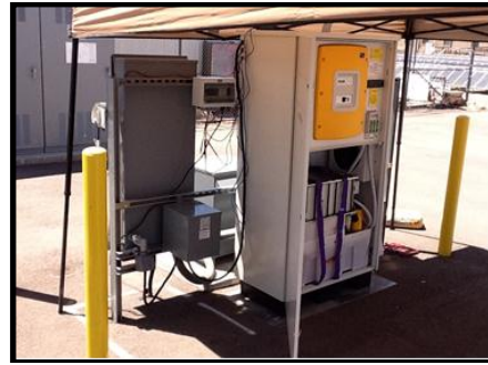
Figure 3: Redflow Zinc-Bromide Battery Module (ZBM) within a System Development Kit (left) and within a demonstration residential unit R510US (right)
