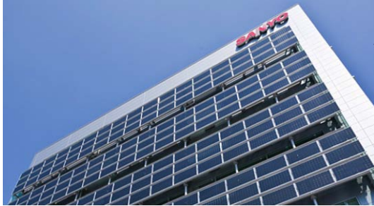
Fig. 5. PV solar deployed vertically on the side surface of a building.
