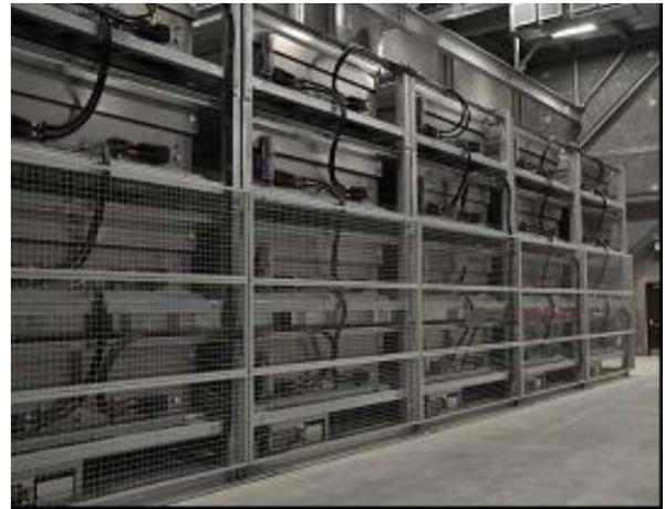
**Fig. 4. NAS battery modules with rack system for ETT/AEP.**
