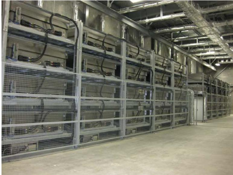
**Figure 4: NAS battery modules with rack system for ETT/AEP**
