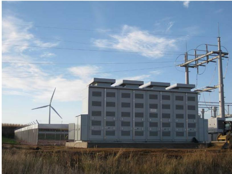
Figure 1: NAS Battery for Xcel Energy.
