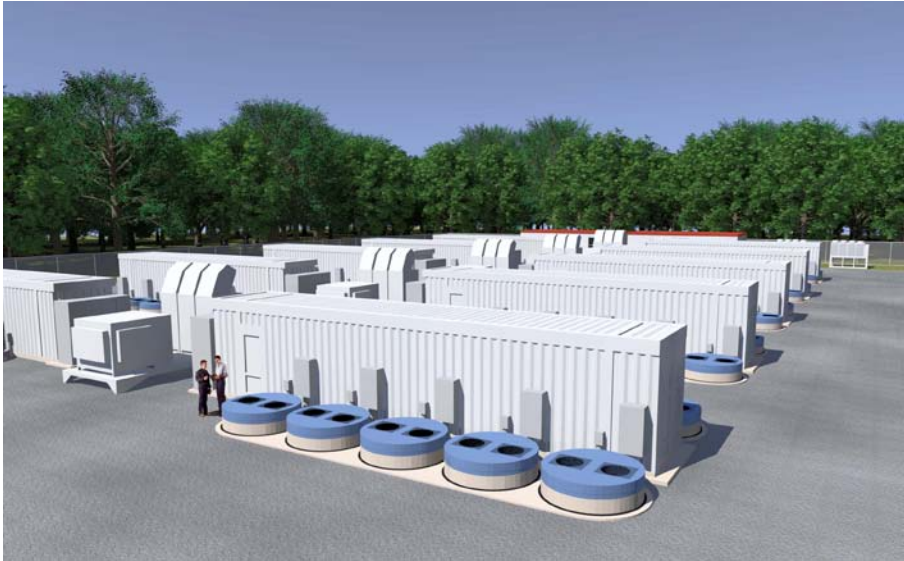
20 MW flywheel regulation plant planned for Stephentown, New York.
