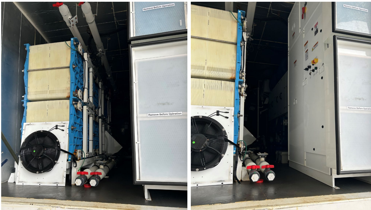
ESS Fe flow battery trailer inside view
