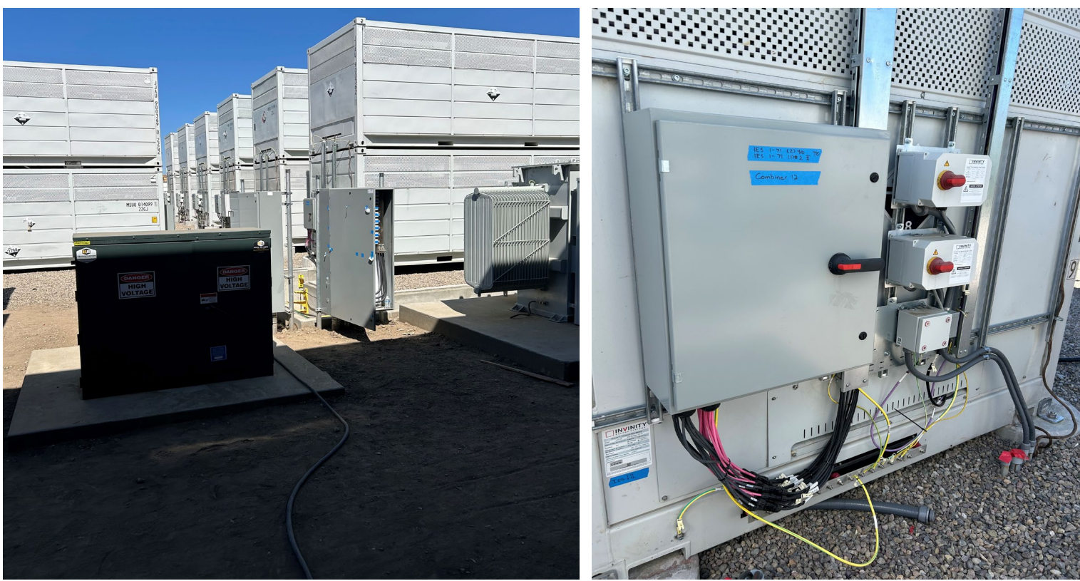
Invinity, V redox flow battery trailers, stacked double deck
