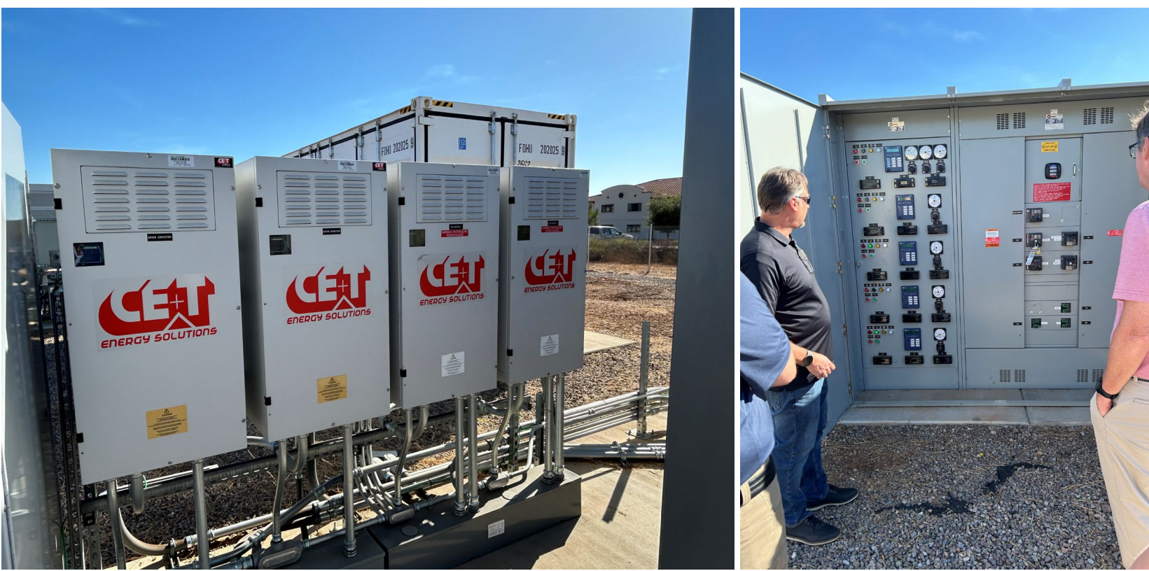
Eaton Supercapacitors at RICU
