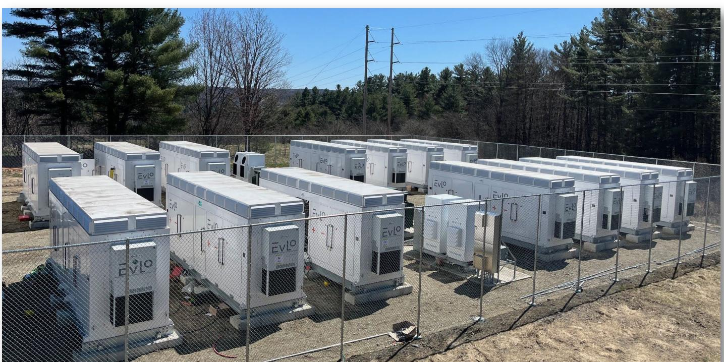
The Troy Battery Energy Storage System (BESS) features advanced technology tailored to address grid challenges. Manufactured by EVLO Energy Storage, the **3MW / 12 MWh, lithium iron phosphate (LFP)** system consists of **16 industrial units equipped** with redundant safety features, including smoke detectors, hydrogen sensors, and natural convection cooling mechanisms. These design elements ensure reliable operation under various conditions while minimizing maintenance requirements.
