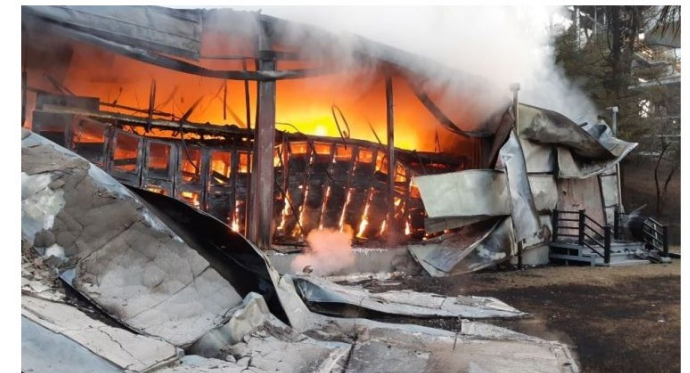
A fire engulfs an energy storage system at a cement plant in Jecheon, North Chungcheong Province, Monday. / Courtesy of North Chungcheong Province Fire Service Headquarters
