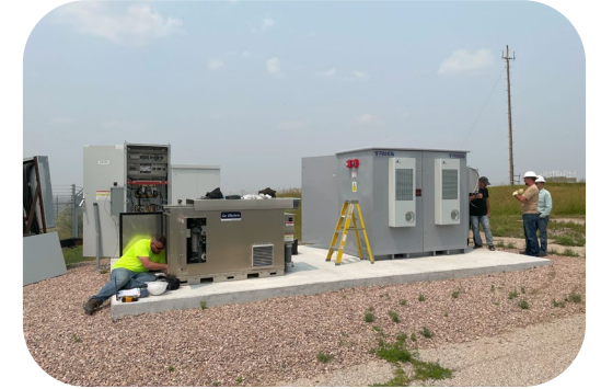
Ellsworth AFB Commissioning
