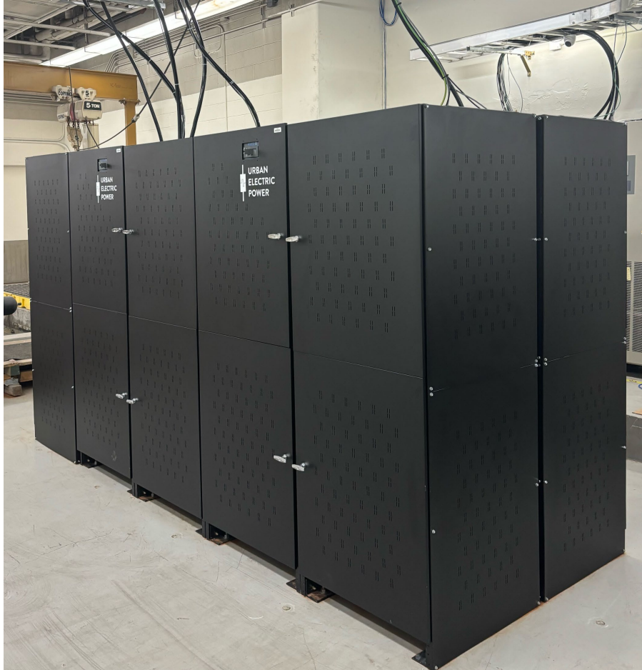
100kW/400kWh system at the City College of New York
