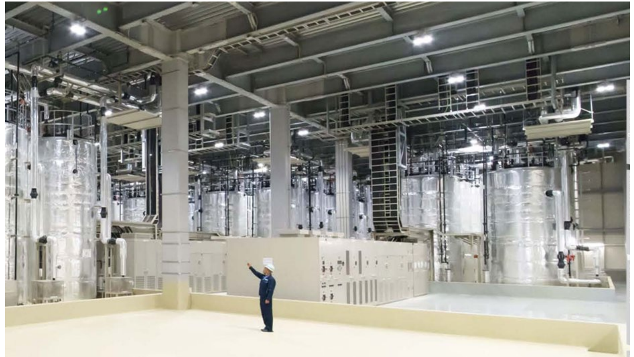
HEPCO Minami-Hayakita Substation
