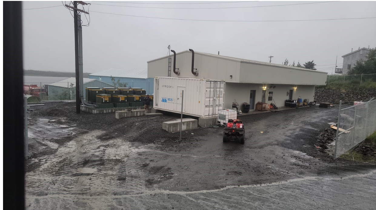
ONE OF TWO MODULES MOUNTED ON SITE AT ST. MARYS POWERPLANT
