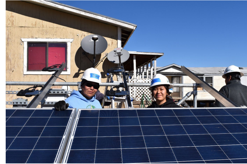
Navajo home being fitted with PV power
