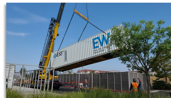
ESS inc. iron flow battery
