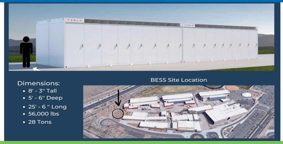
Largest Tesla installation in New Mexico – 721 kW / 2884 kWh
