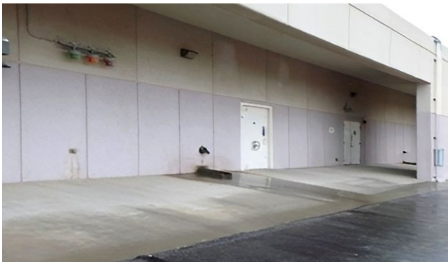
SAFER SPACE — The Explosive Technologies group overhauled an outdoor area, rehoming unneeded items and transforming it into a safer space.
