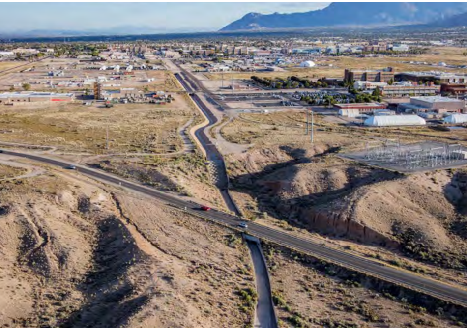
CLEANER STREAMS — Stormwater drains from the Labs at the Albuquerque site into a concrete channel that discharges into the Tijeras Arroyo.
