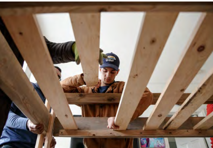
BUILD A BED — Communications intern Michael Shaikh lays slats in a bunk bed. Photo by Spencer Toy
