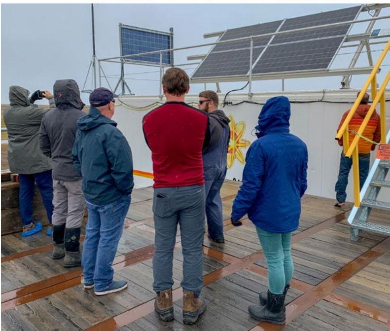
GATHERING DATA — The group from Infrastructure and Security Operations observed the photovoltaic system installed atop a shipping container at Oliktok Point.
