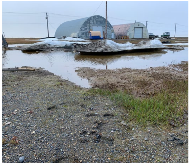
COOLER CLIMES — Melting snow and ice can present challenges to accessing some of Sandia's Arctic facilities. Photo by Matt Cattaneo
