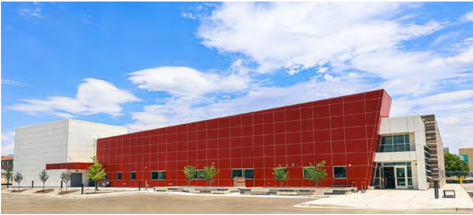
STYLISH STOREFRONT — Sandia's new Emergency Operations Center will house NNSA and Labs emergency management staff offices. Photo by Lonnie Anderson
