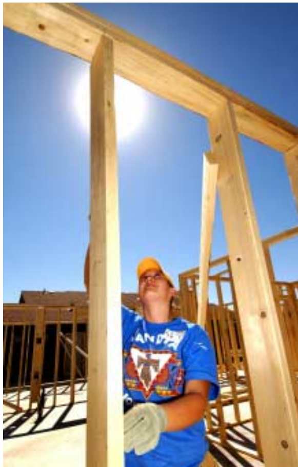
VIRGINIA VIGIL (6863) aligns a newly framed wall.
