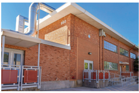
Access ramps and an elevator bank were added to the east end of the Environmental Test Lab (Building 860) to comply with access requirements while preserving the historic design of the building. Photo by Randy Montoya
