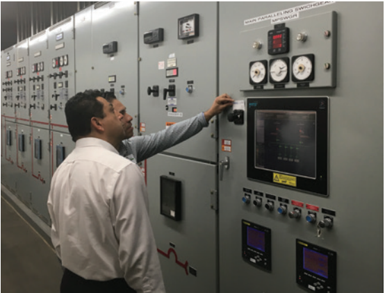
SWITCH REVIEW — Sandia employees inspect a bank of switchgear, which are used to monitor, control and protect different power assets that make up a microgrid.
