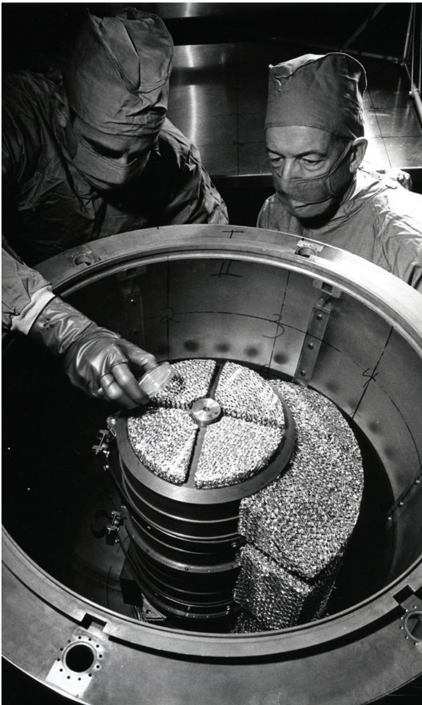
CLEAN SLATE — Ed Powers of NASA, left, and Sandian Vernon Arnold inspect the sterilization of an interplanetary lander in this 1965 photo.
