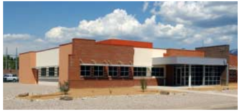
. . . BLDG. 753 TODAY, occupied by the Integrated Studies and Support Group of Nuclear Weapons Program Integration Center 9700.
