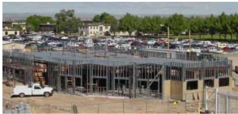
BLDG. 753 under construction in May, and . . .
