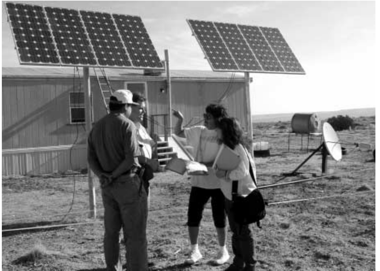
AT HOME WITH PHOTOVOLTAIC SYSTEMS — Miriam Hilborn, second from right, talks to visitors from the National Indigenous Institute in Mexico about the photovoltaic system she and her husband Duane use to electrify their house on Laguna Pueblo lands. Their home is totally powered by a photovoltaic/wind system.
