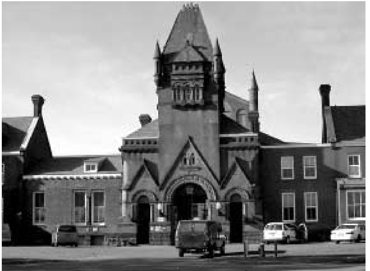
TO HELP DEVELOP a security vulnerability assessment methodology useful to prison officials, Sandia and the State of Pennsylvania Department of Corrections conducted a pilot assessment at Huntingdon State Correctional Institution, seen here.
