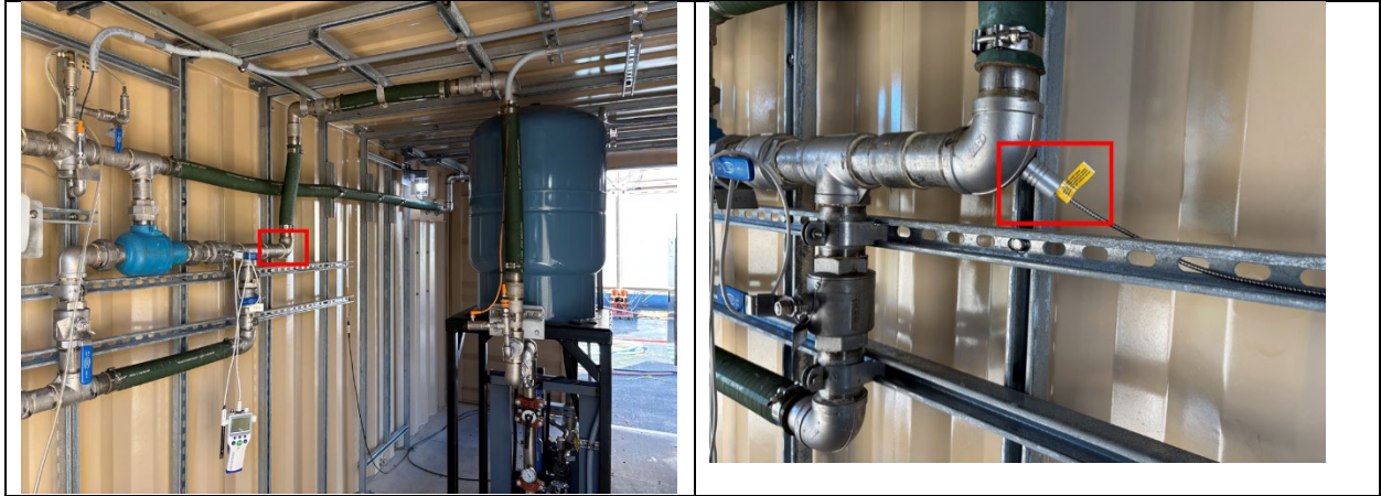
Figure 12. Temperature Sensing Placement
