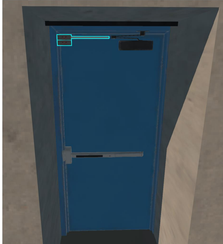
Figure 11. Reactor Building Balanced Magnetic Switches
