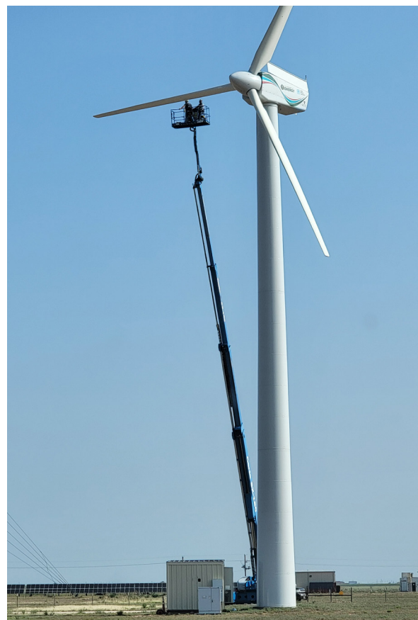
Aerodynamic sensor installation on one of the SWiFT Turbines (Photo by Johnny Luevano).
