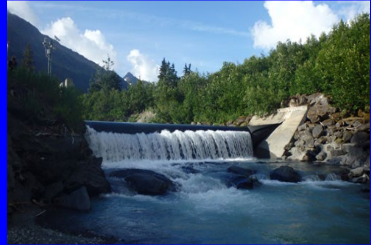
6MW Run of River Hydro Power
