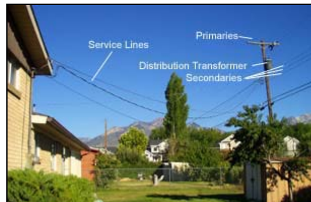
Figure 23: Household Service Line Drop from Distribution Line
