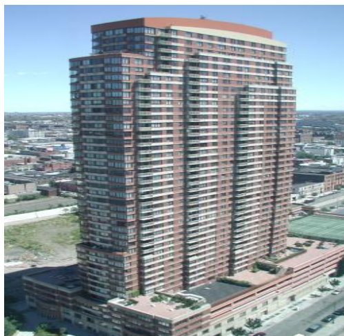
Figure 4.4. Arista Multi-Story Building, NYC
