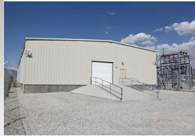
Dedicated ESS Building
