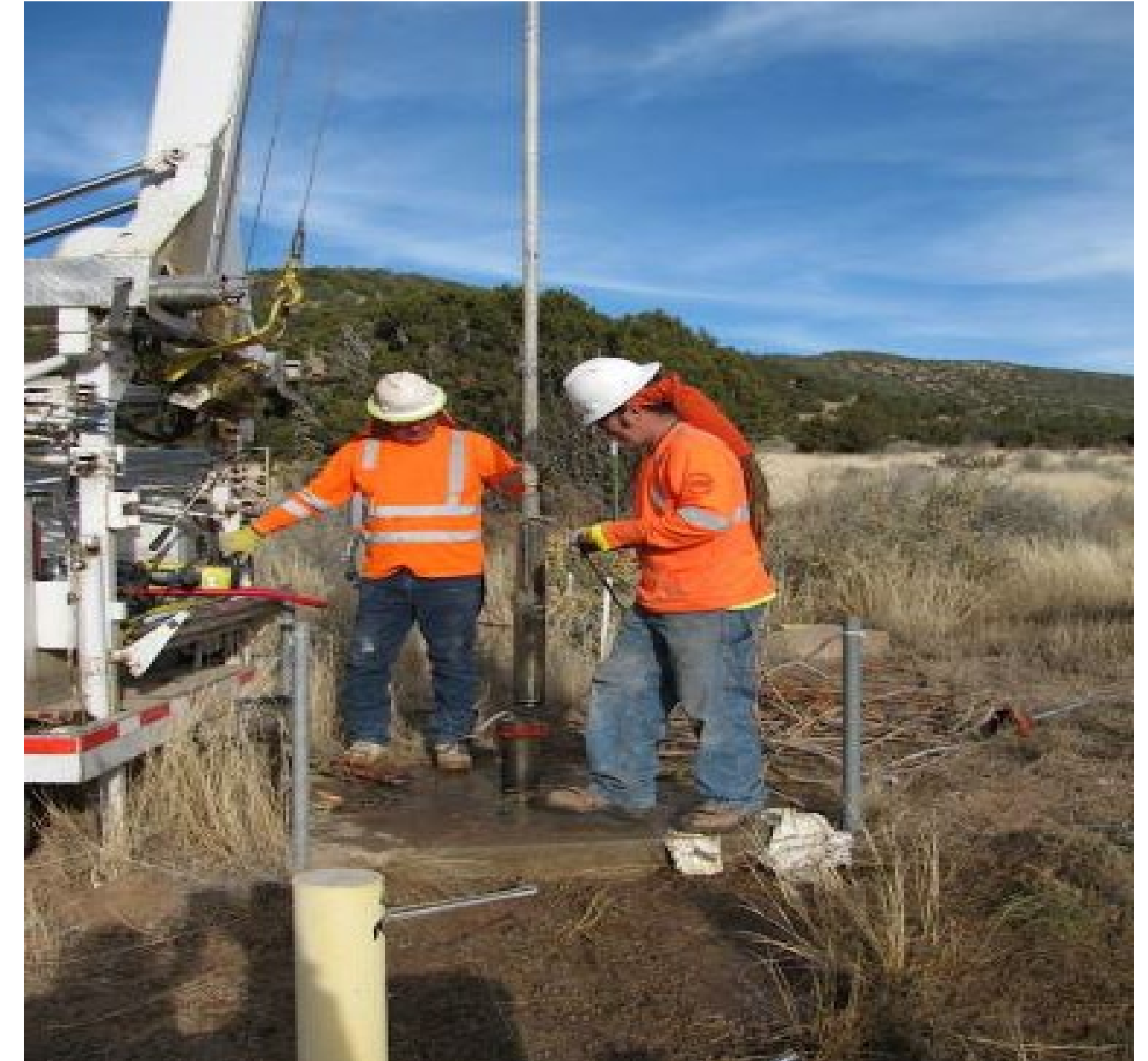
Drilling at Burn Site
