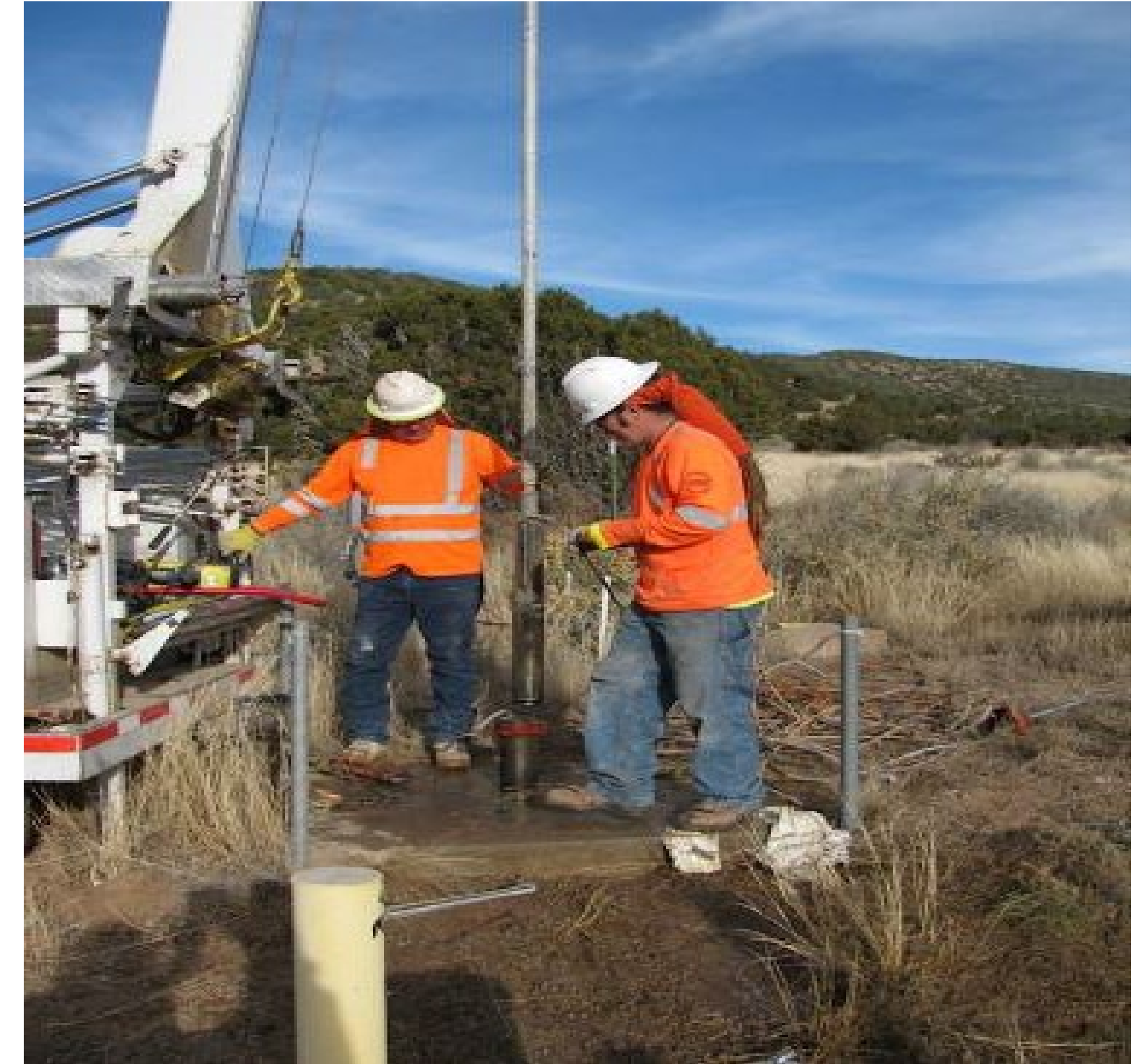
Drilling at Burn Site
