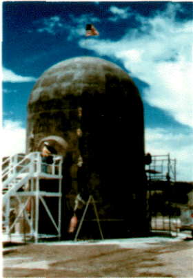
THE 1/6-SCALE REINFORCED CONCRETE MODEL
