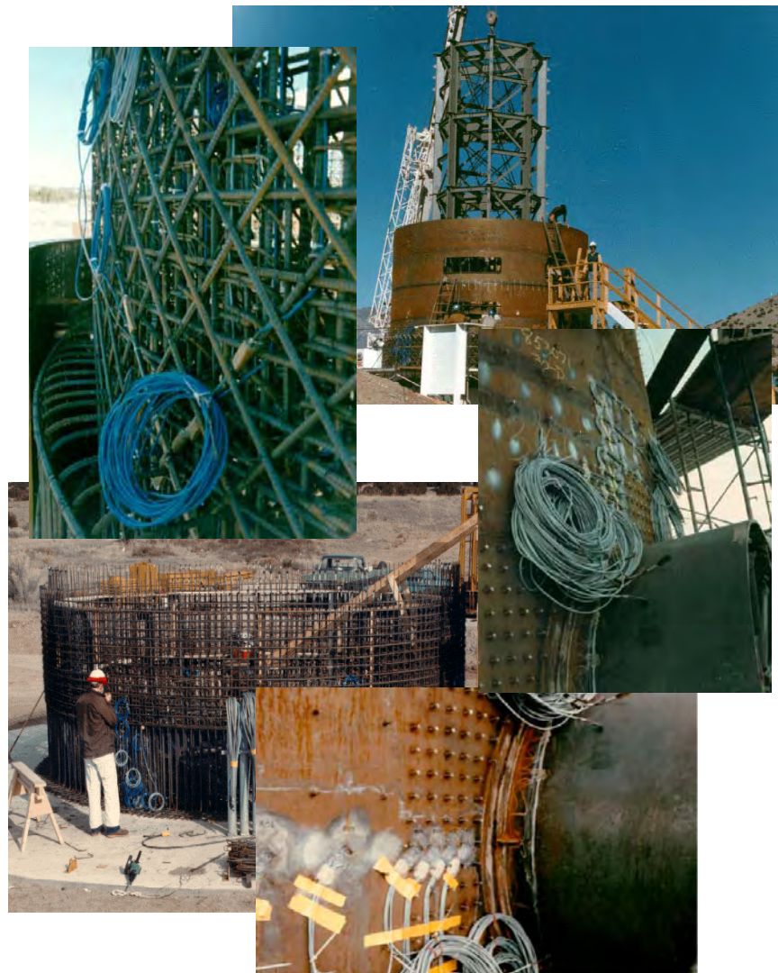
Figure 38 1:6-Scale Reinforced Concrete Containment Model Construction
