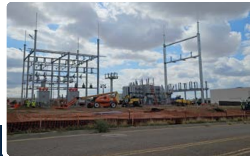
PNM's Sandia Energy Battery Storage System under construction.
