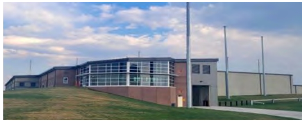
A new facility at F.E. Warren Air Force Base, where Sandia assisted with government acceptance testing. (Photo courtesy of the U.S. Army Corps of Engineers)
