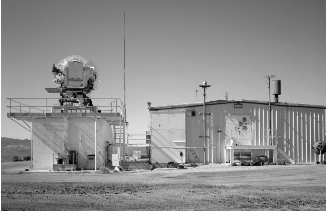
Buildings 24-00 (Support Radar Antenna Building) and 24-01 (Support Radar Lab Building), contributing resources to the SNL/TTR historic district (Photo taken on August 11, 2004, by Joseph M. Bonaguidi)
