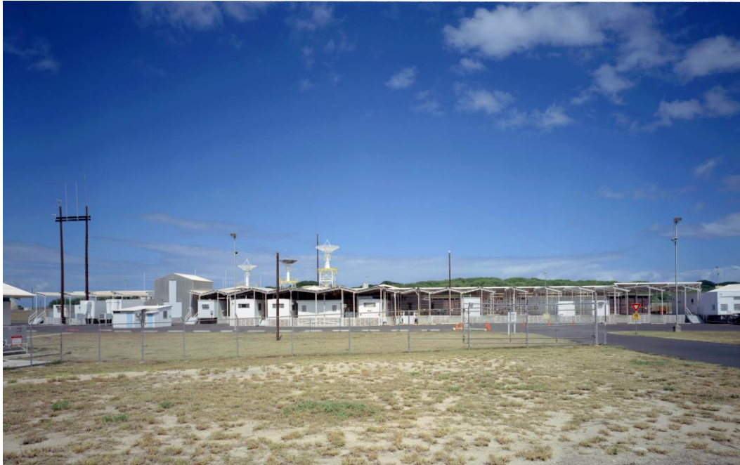
Administrative compound, Kaua'i Test Facility (Photo by Joseph M. Bonaguidi)
