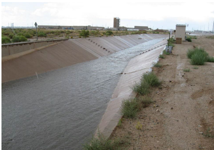
Stormwater drainage channel to Tijeras Arroyo
