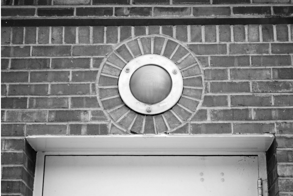
Exterior light set in a brick sunburst design on historic Building 840, one of the early buildings designed by New Mexico architect W. C Kruger’s firm
