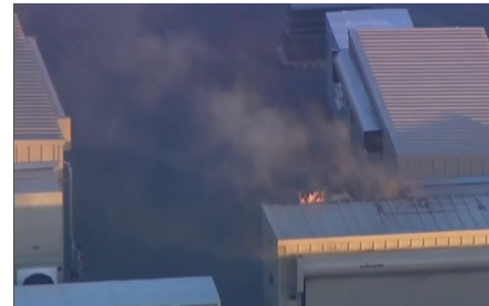
2023 Battery Storage Facility
