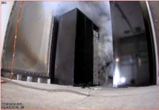
Smoke accumulation [TR + 00:00:31]
