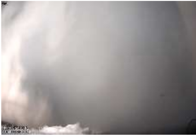
Novec 1230 discharge [TR + 00:00:58]
